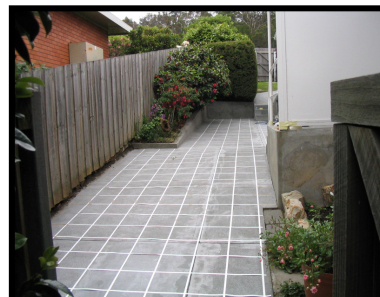
Picture Left: Primer Plus applied to prepared concrete.
