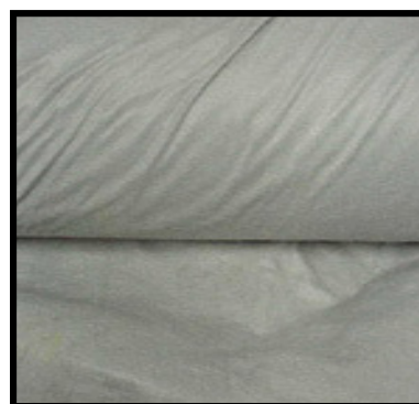
Top Picture: Poly cloth and Watershield C applied to prepared concrete.
